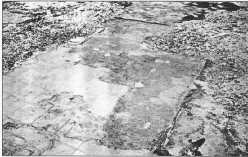
If spalling has a pattern, and if there is unusual, higher thermal dynamic activity than indicated by the normal fire load, then spalling should be considered a possible indicator of arson.
