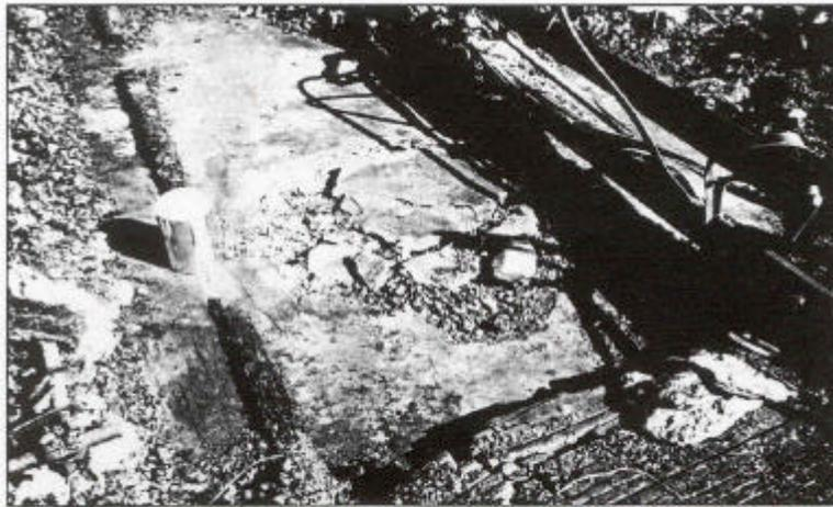
Some of the most dramatic examples of spalling are thought to be caused by entrapped moisture at very high temperatures. Some investigators believe this type of spalling can occur deep in concrete and produce larger, thicker chips, but even that generalization on this subject is very difficult at best.
