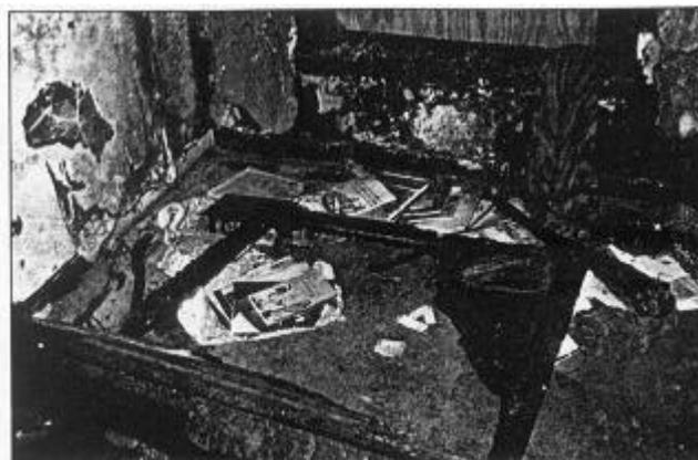
Burning curtains dropped to the floor causing a hot spot which was incorrectly interpreted as a separate and unconnected origin. (This photo is in the same structure as photo on page 4).
